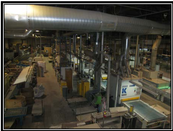
Plant View from Mezzanine
