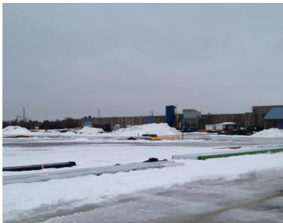
Storage Yard on East Side of Building
