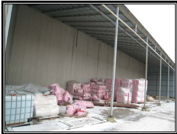
Unenclosed Rear Storage
