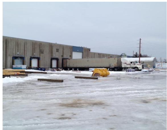
West Side Storage and Shipping Docks
